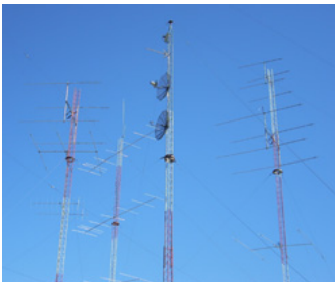
The 7th place Multi-Op KB0HH contest station in northwest Oklahoma has four rotating towers: 6 meters, 2 meters, 222/432 MHz, and microwave with multi-beam arrays on 50, 144, 222, and 432 MHz and parabolic antennas for 1296, 902, and 2304 MHz.
